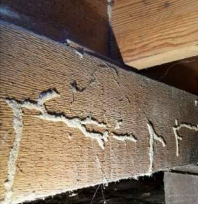
Center beam in Crawl space
