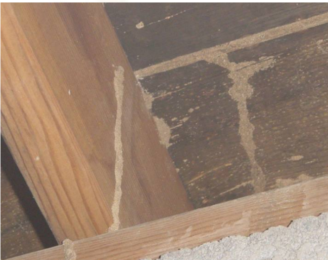
Back wall of the crawl sapce
