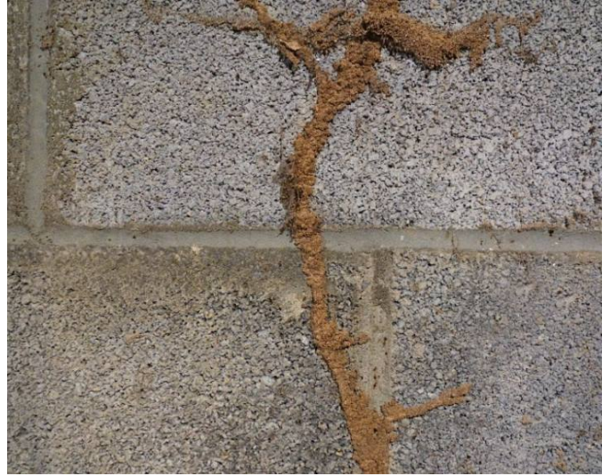
Back wall of crawl space
