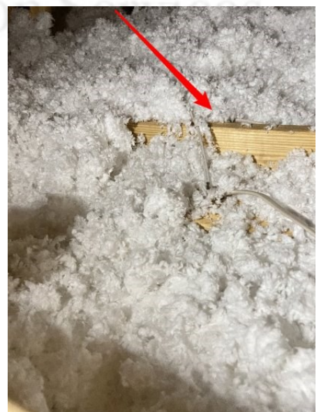
Bottom chord of roof truss is 5 1/2 inches high.
