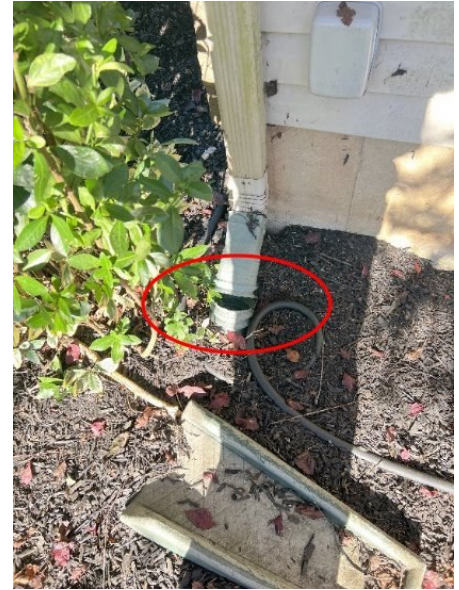
Right front corner
