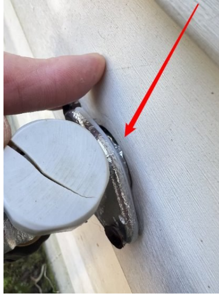
Exterior spigot left side of house
