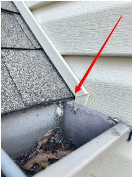
Option 1 & 2 for kick out or diverter flashing
