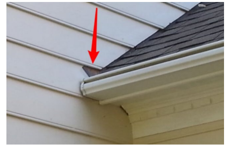
Option 3 for diverter flashing
