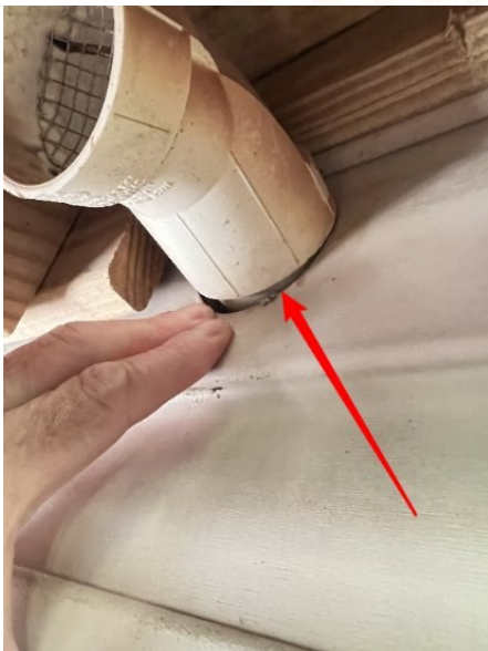
Rear of house under the deck
