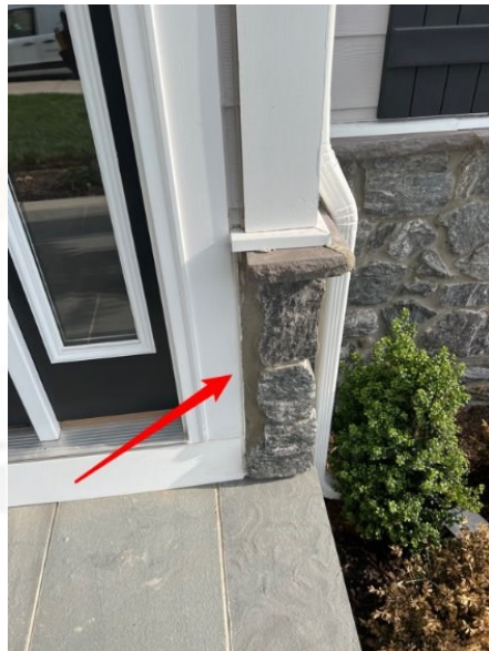
additional caulk backer needs to be installed where there are gaps
