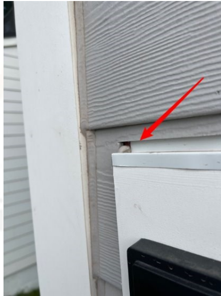
no caulking behind the vent
