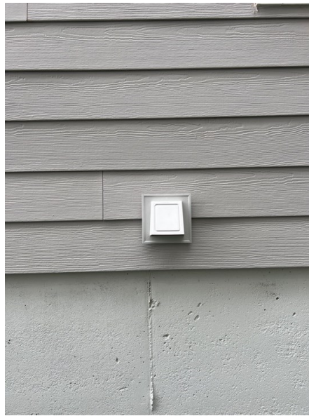
no caulking behind the vent
