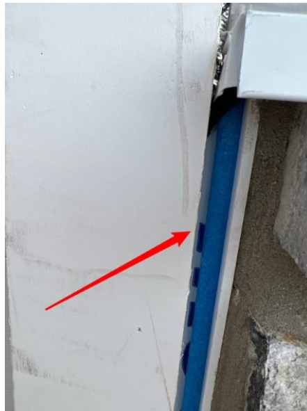
additional caulk backer needs to be installed where there are gaps
