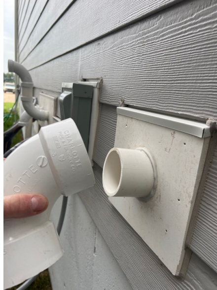
The elbow should be glued in place
