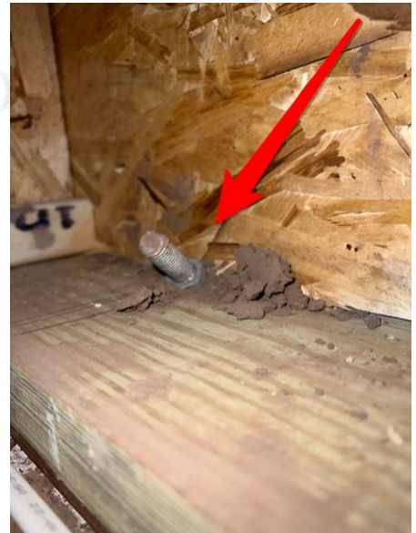
Left foundation wall
