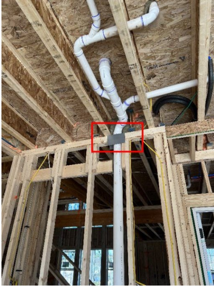
Rear wall of the garage
