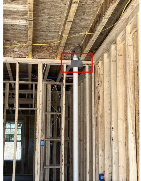
Rear wall of the garage
