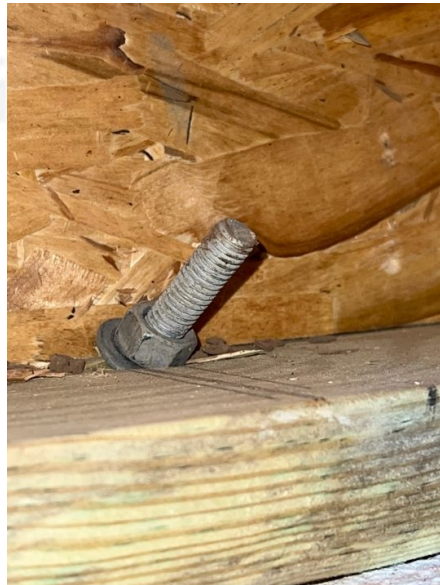
Left foundation wall
