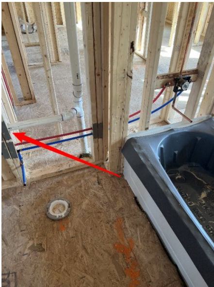
second floor center bathroom
