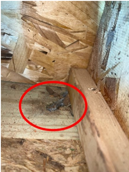
Left foundation wall
