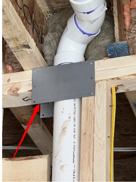
Steel plate not adequate
