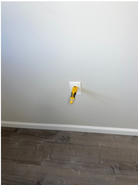
Left wall of left front room in the basement.
