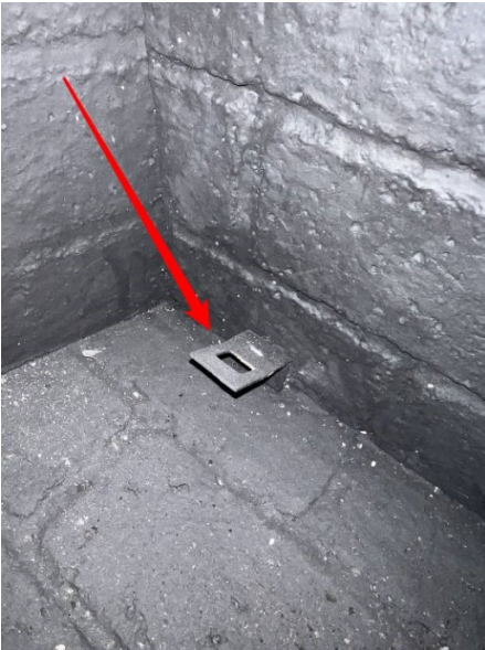
log holder should fit in brackets
