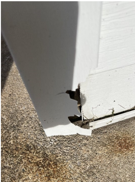
Bottom corner of the chimney
