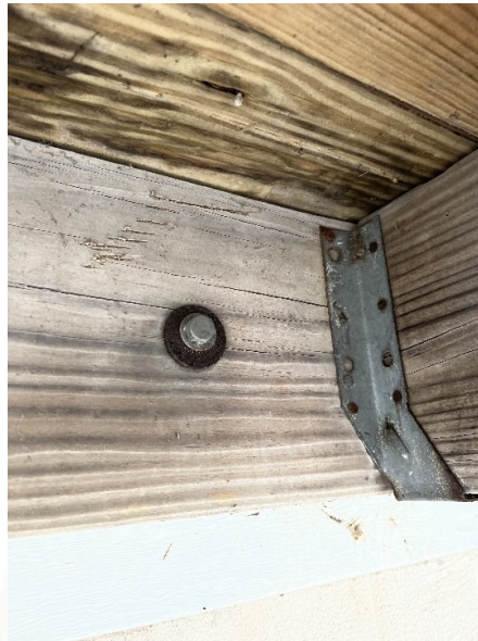
Flashing needed to prevent water from running behind the ledger board
