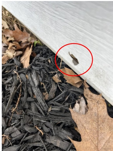
Left front of the house
