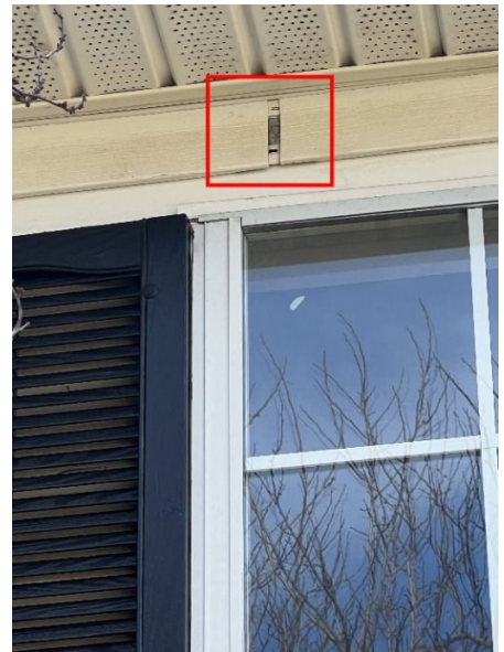
Front of the house above the right second floor window.
