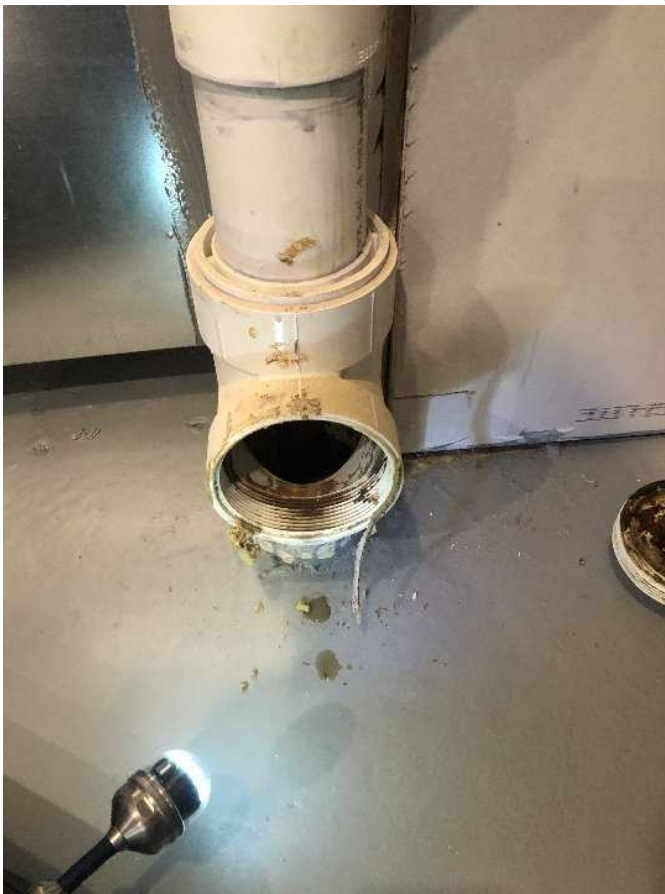
Camera access through interior clean out
