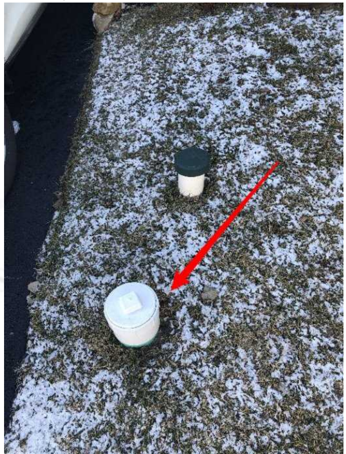
Camera accessed through the exterior vent
